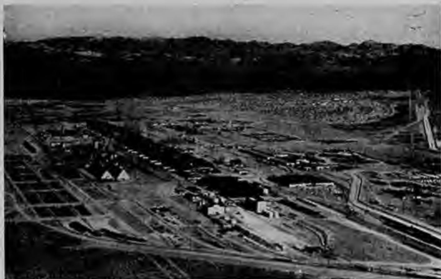
Fig. 3.—An aerial view of the large plant designed and built by Magnesium Elektron Limited for the United States Government. This plant, designed to produce 50,000 tons per annum, produced its first metal ten months from the day the ground was broken.
